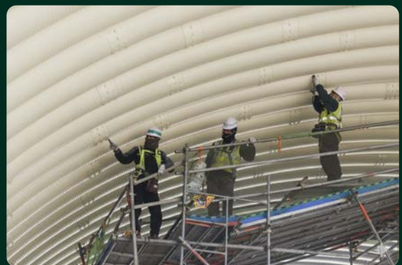
WonderArch Method (Assembly after electro-coating)
